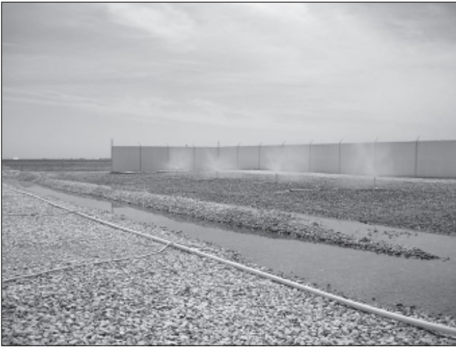
Red Rock Ranch solar evaporation drainage water system.
