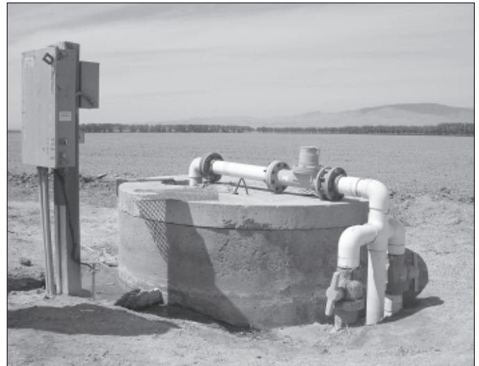
This drainage sump at Red Rock Ranch will be used to collect monitoring data.
